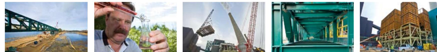
While the environmental retrofit of Unit 3 has been the focal point of Boswell improvements in 2008-09, other major construction was underway at Minnesota Power's largest power plant. A new bridge bearing sealed tubes to move dry ash from the new Unit 3 baghouse as well as coal ash from two other Boswell generating units was built. In the future, ash will be transported by these tubes in dry form.
