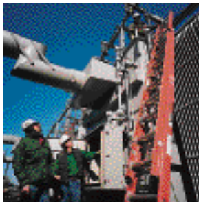
Strengthening successful relationships with its industrial customers is one of the key moves highlighting MP Electric's strategic update. At Inland Steel Mining Company, Reed Rosandich and Larry Tokarczyk of MP Electric (left and top) work with Inland's Marty Zuponic
