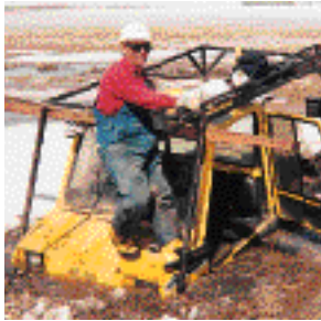
His all-terrain vehicle headlight-deep in mud, MP Electric lineman Carl Thesing teamed with more than 50 MP Electric workers last winter to help restore power along the Minnesota-North Dakota line after catastrophic storms and flooding.
